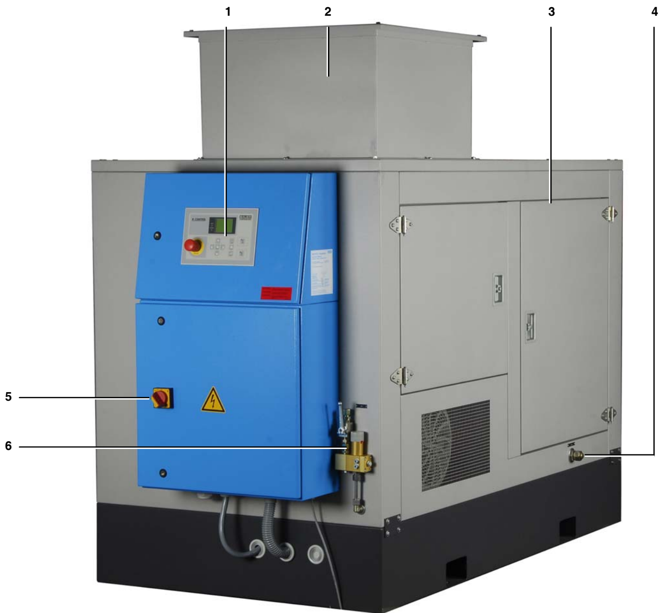
Fig. 8 Industrial compressor unit K22-K23, Super-Silent version
